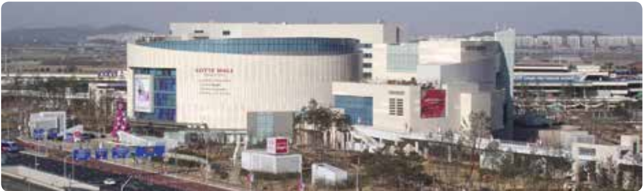
Gimpo Sky Park in which the Distributed Geothermal Energy Use System is applied
