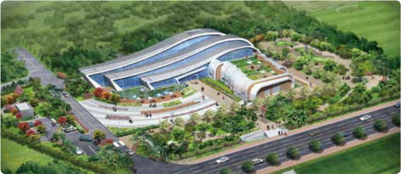
Sewage Water Reuse Facility in Pohang
